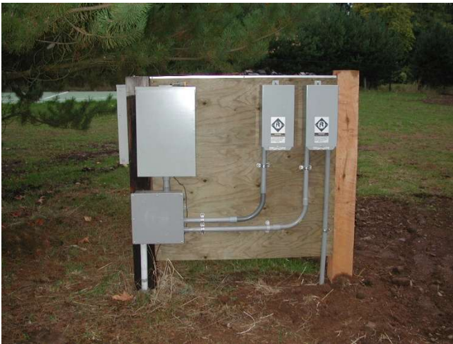
Well head electrical panel
