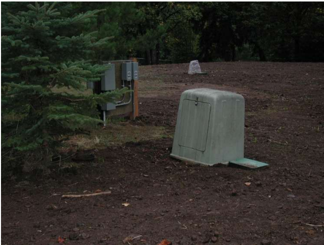
Well head electrical panel
