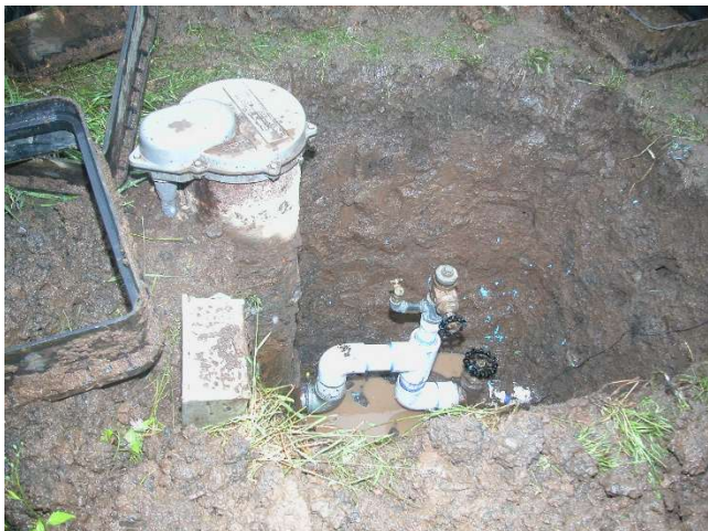
upgrade to pit less adapter
