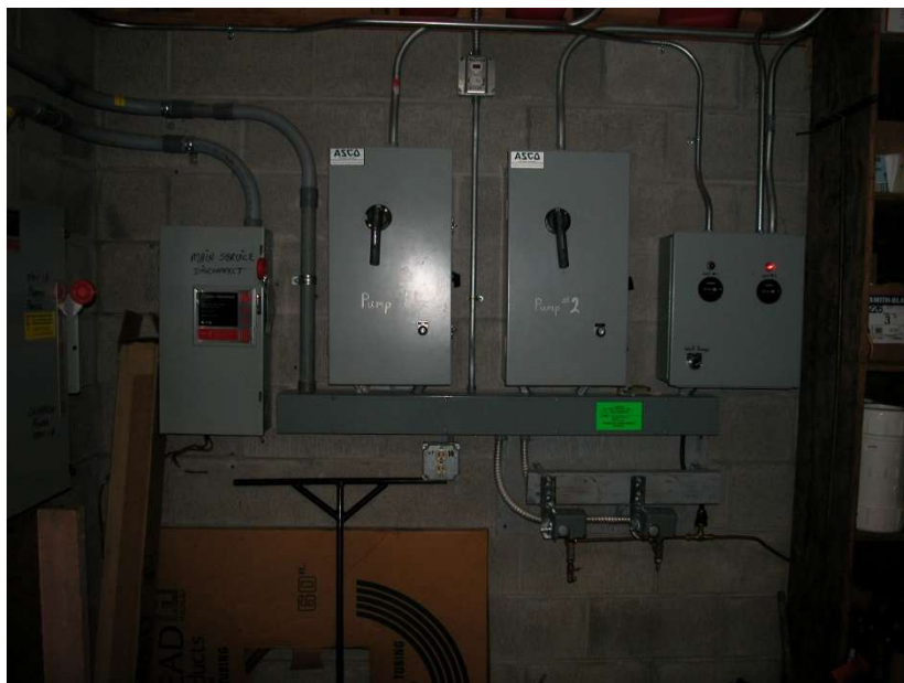
Well Pump Controllers & Switching Circuit
