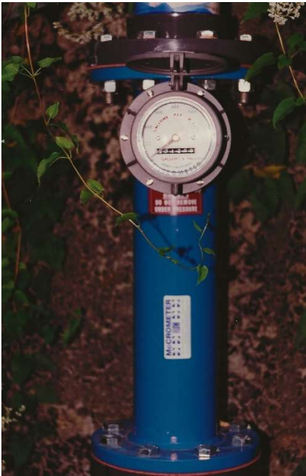
Well flow meter installed
