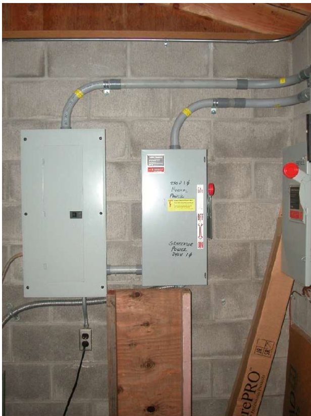
Breaker Panel & Transfer Switch
